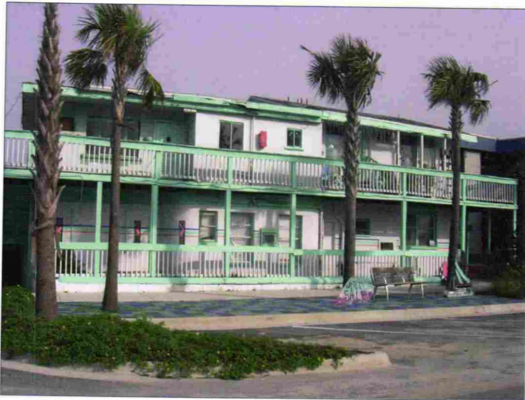
Figure 4.100 Resource 8SJ3937, facing northeast.
