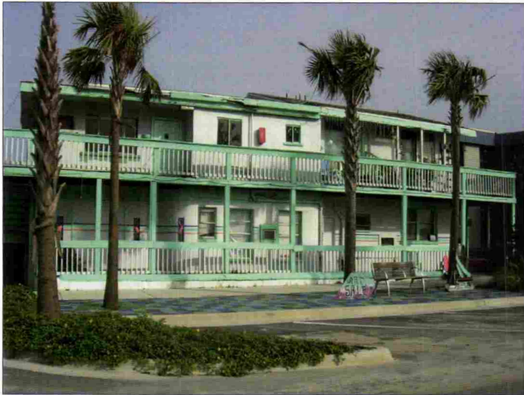
Figure 4.98 Resource 8SJ3937, facing northeast.
