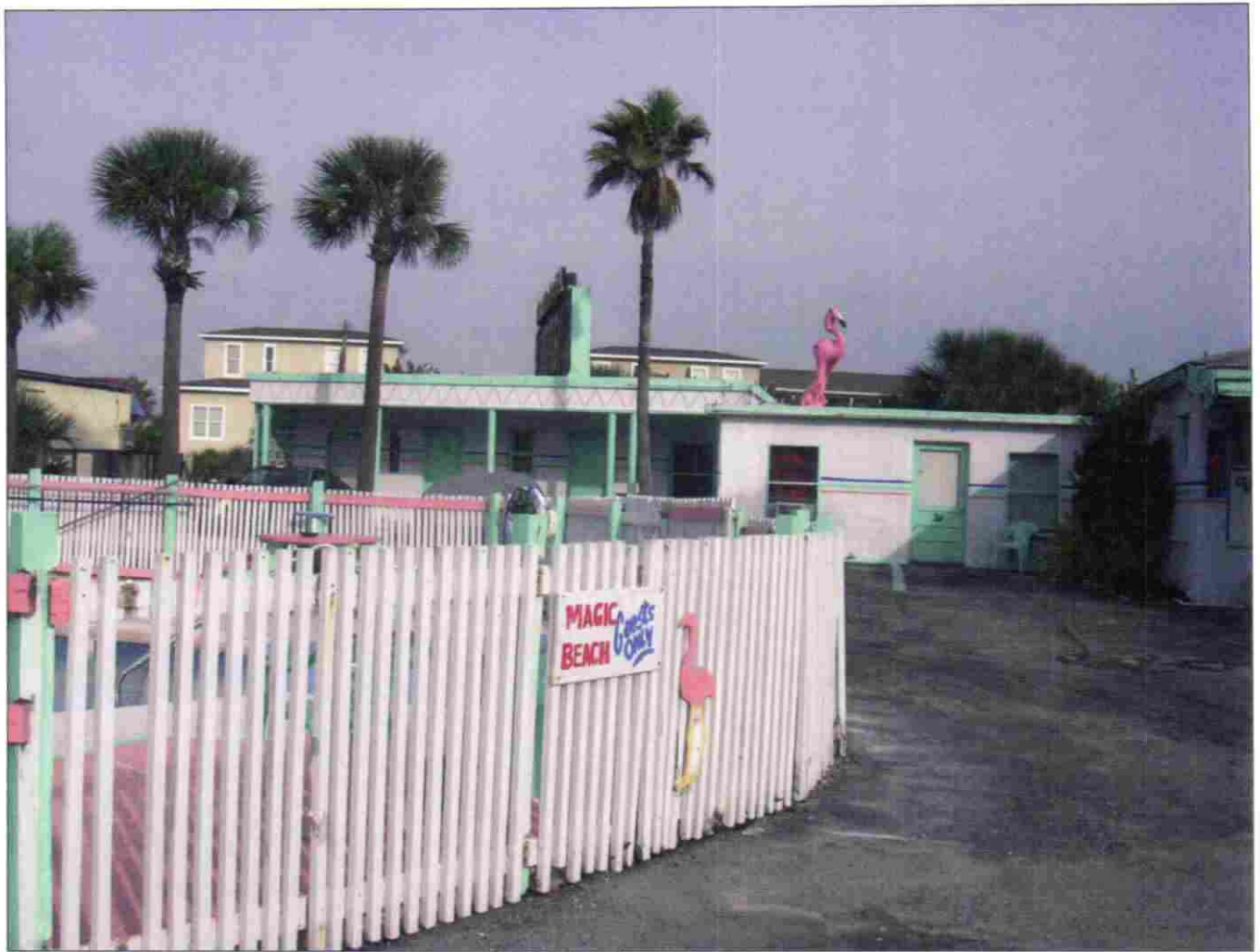
Figure 4.101 Resource 8SJ3937, motel pool view, facing northwest.
