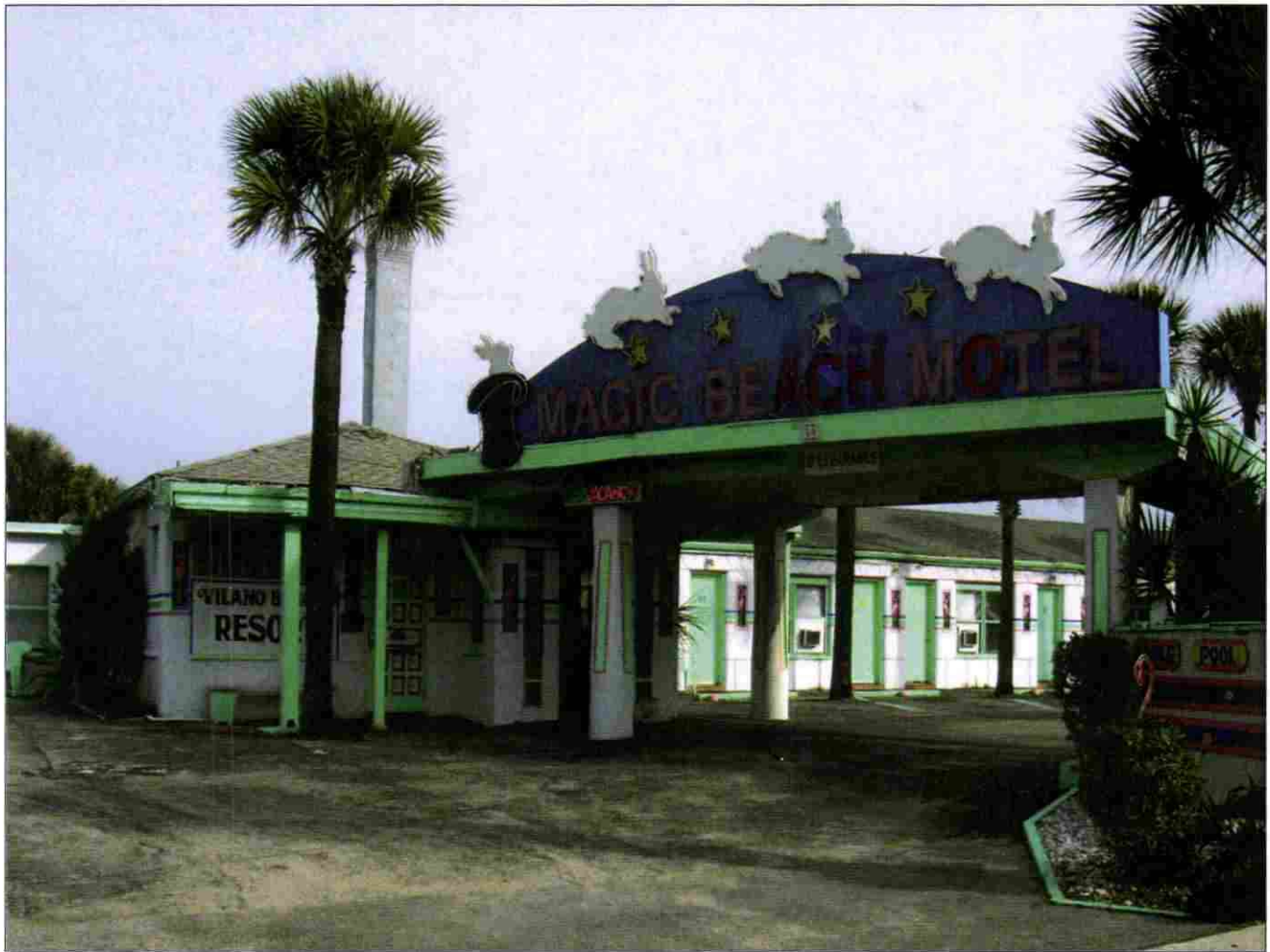
Figure 4.96 Resource 8SJ3937, facing northeast.
