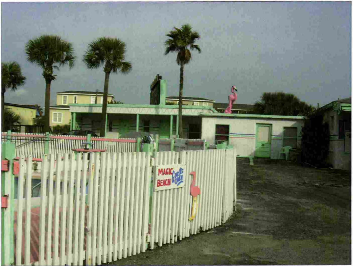
Figure 4.99 Resource 8SJ3937, motel pool view, facing northwest.
