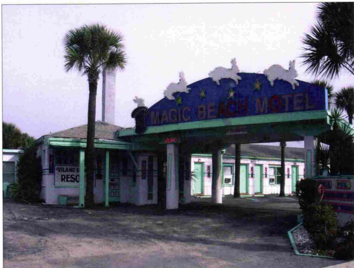
Figure 4.98 Resource 8SJ3937, facing northeast.
