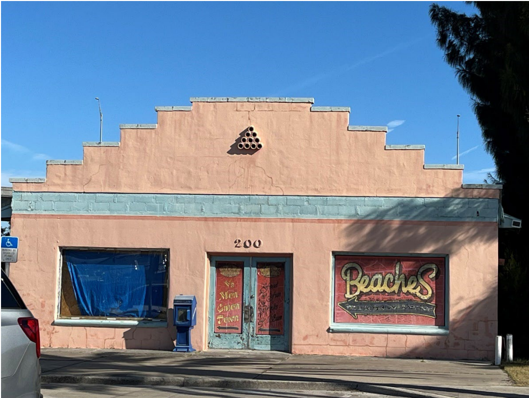
Other structures along Vilano Beach Main Street
