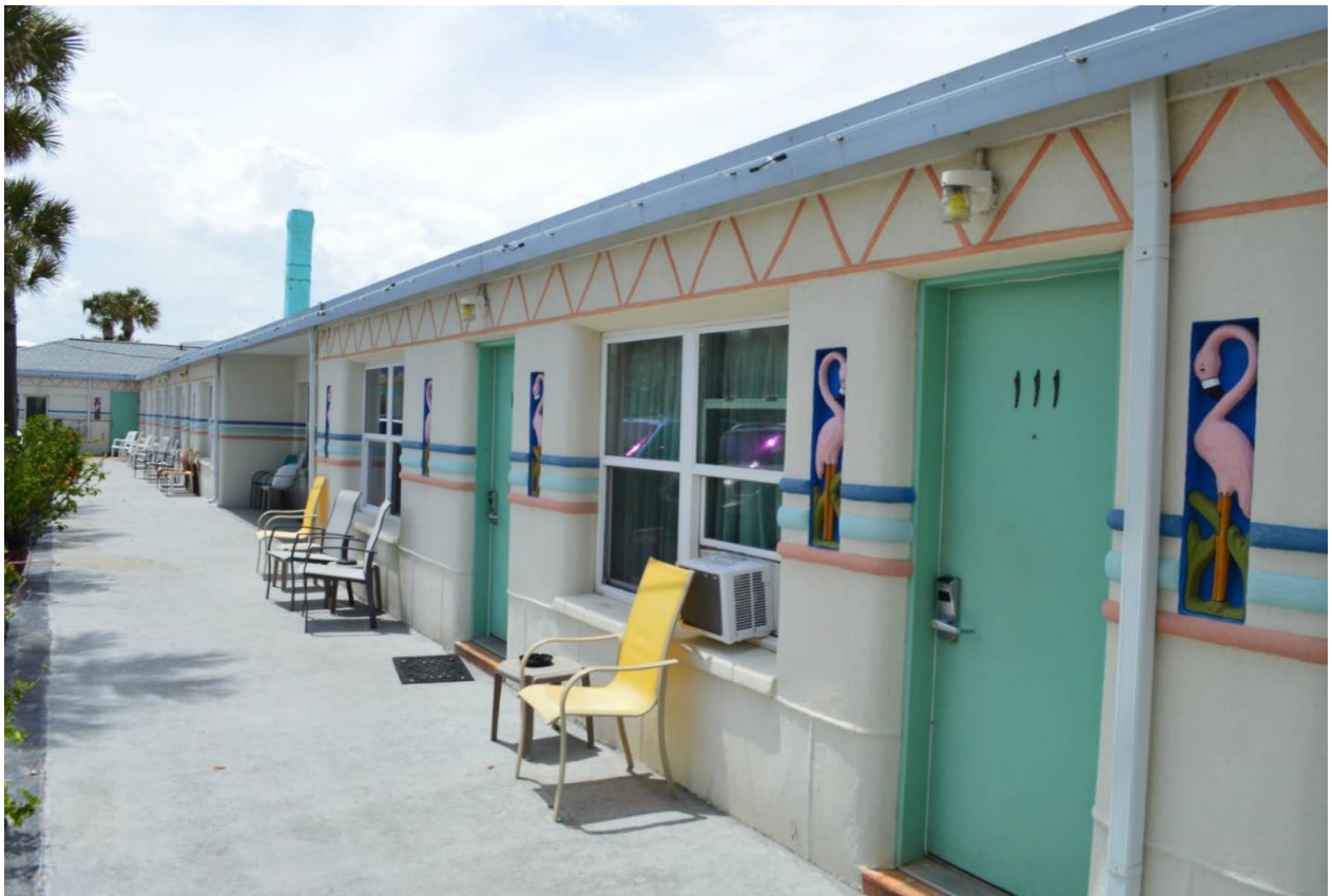
FIGURE 4: MODERNE DETAILING, EAST WING
