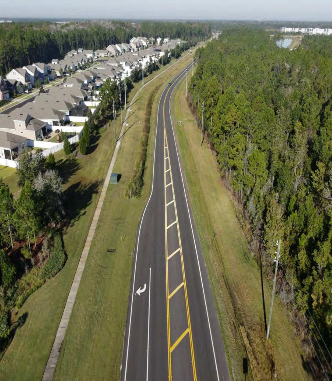
Old CR 210 & Twin Creeks Drive Pavement Management Project
