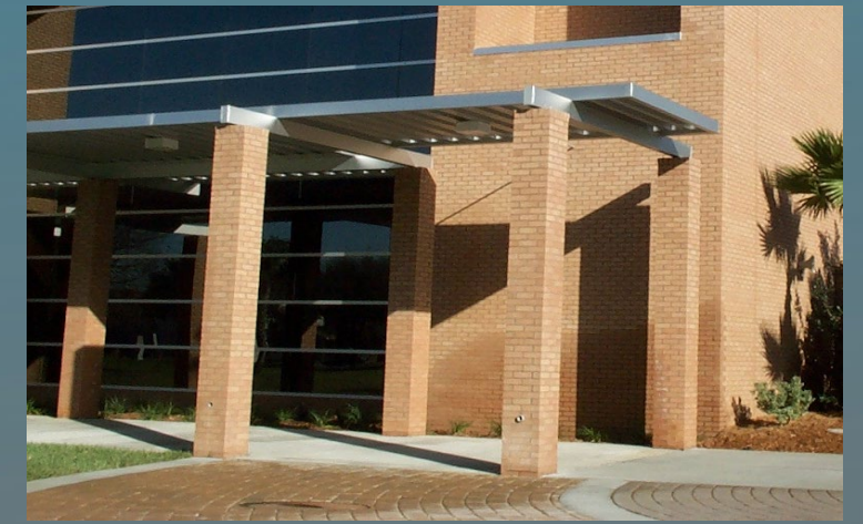
4. PREFABRICATED METAL CANOPY
