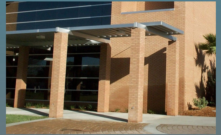
4. PREFABRICATED METAL CANOPY
