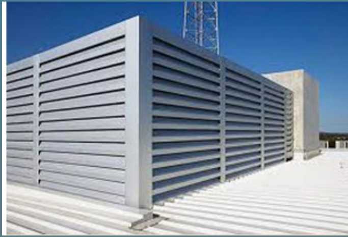
1. METAL MECHANICAL SCREEN
