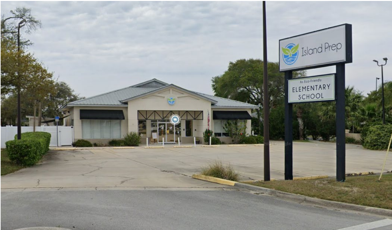
Existing Island Prep Building at 4001 A1A South:
