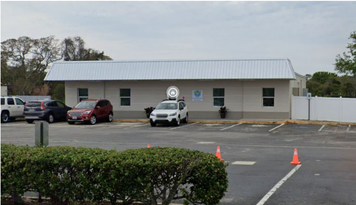
Existing Island Prep Building at 4035 A1A South:
