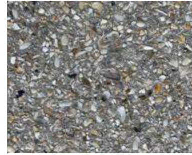
3. Exterior pavement Exposed aggregate coquina
