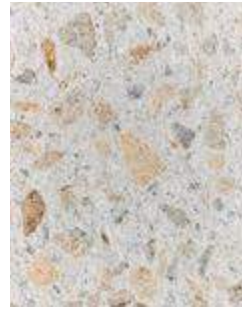
2. Exterior pavement Exposed aggregate conc.
