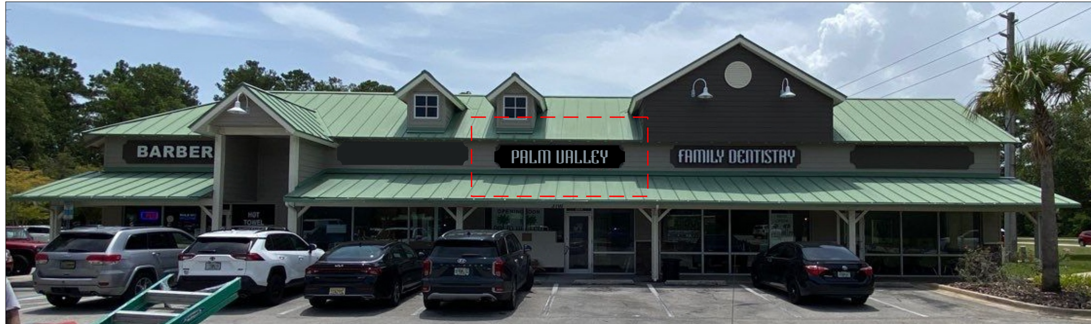
Photo Overlay - Internally Illuminated Letters
