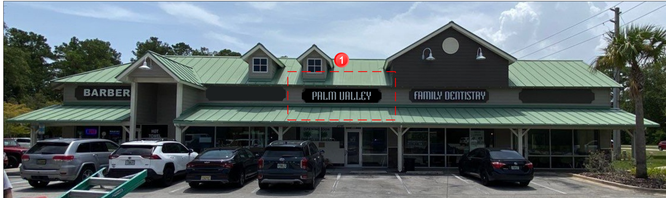
Photo Overlay - Internally Illuminated Letters
