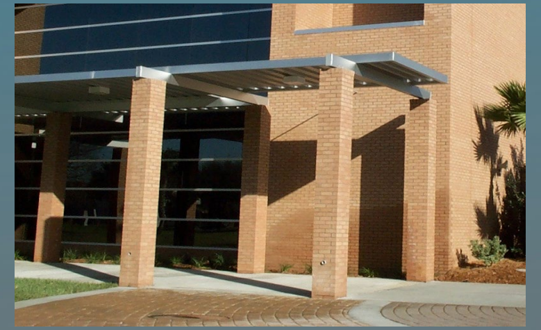
4. PREFABRICATED METAL CANOPY
