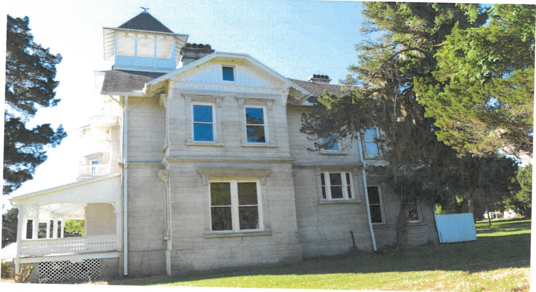
• PHOTO 11: NORTH FAÇADE, BELVEDERE, EASTLAKE AND Poured CONCRETE DETAILING, FACING SOUTH
