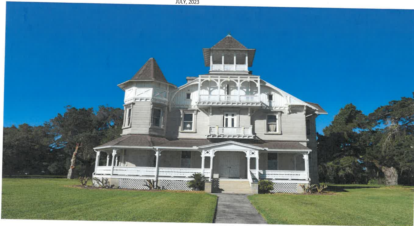
• PHOTO 4: MAIN (EAST) FAÇADE, FACING WEST.
