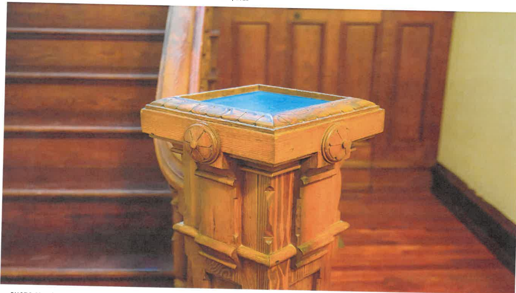
• PHOTO 27: 1 ST FLOOR, NEWEL POST, MAIN STAIR, FACING NORTH
