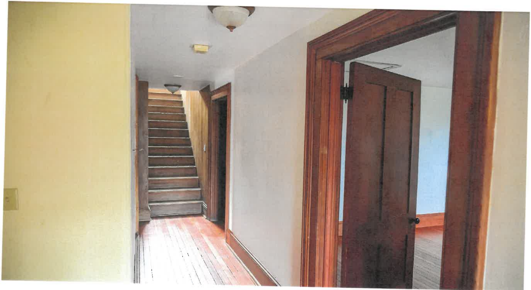
• PHOTO 38: 3RD FLOOR, HALL, STAIR TO BELVEDERE , FACING EAST
