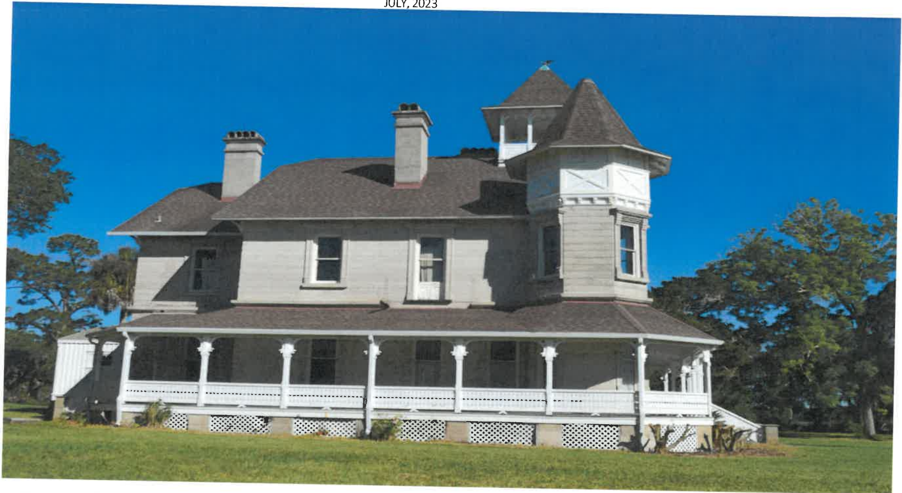
• PHOTO 9: SOUTH FACADE, FACING NORTH
