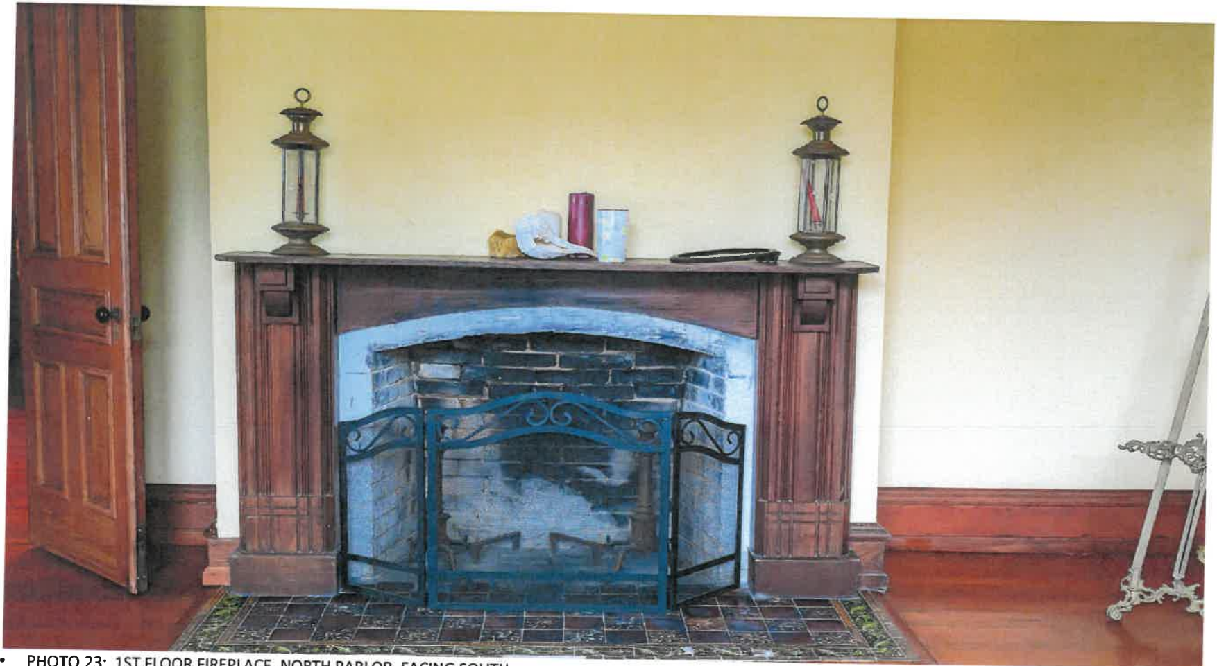
• PHOTO 23: 1ST FLOOR FIREPLACE, NORTH PARLOR, FACING SOUTH
