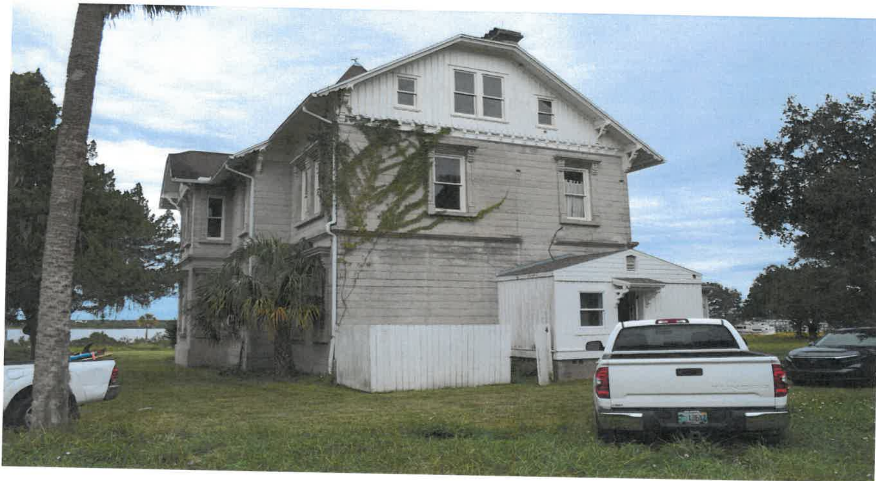
• PHOTO 15: WEST FACADE, FACING EAST
