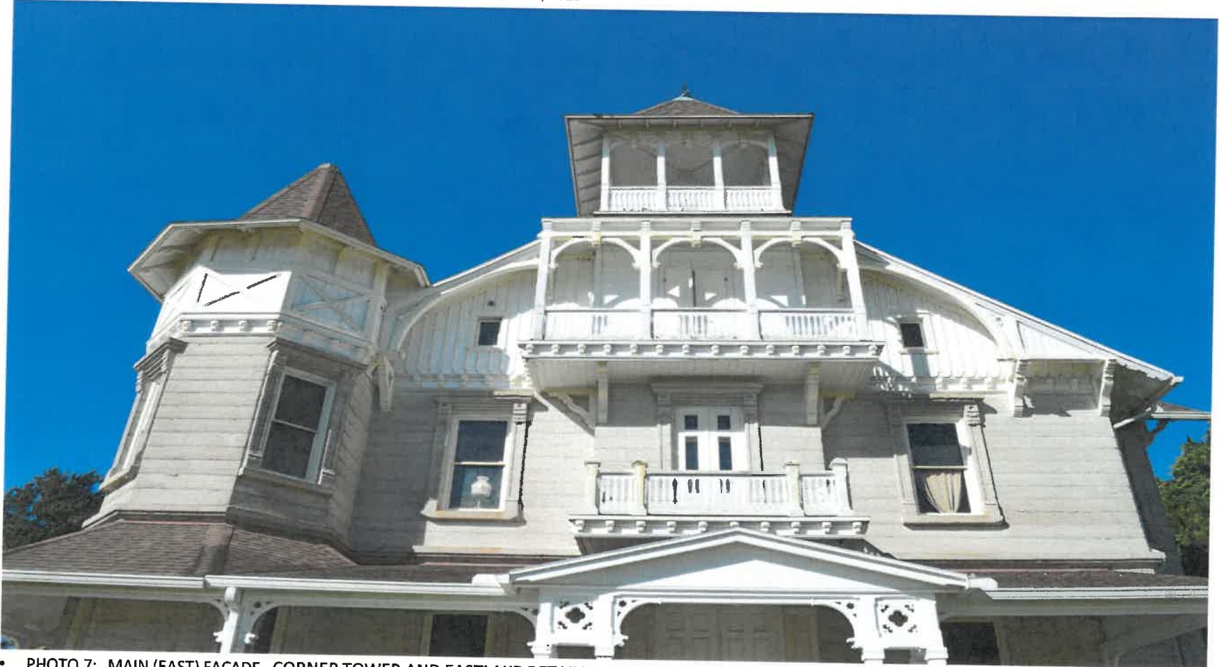
• PHOTO 7: MAIN (EAST) FAÇADE , CORNER TOWER AND EASTLAKE DETAILING, FACING WEST
