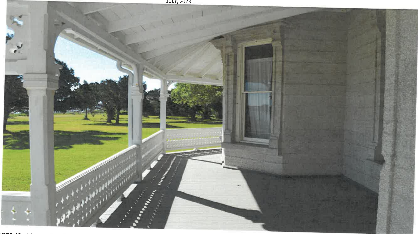
• PHOTO 13: MAIN ENTRANCE/PORCH, POURED CONCRETE DETAILING, FACING SOUTH
