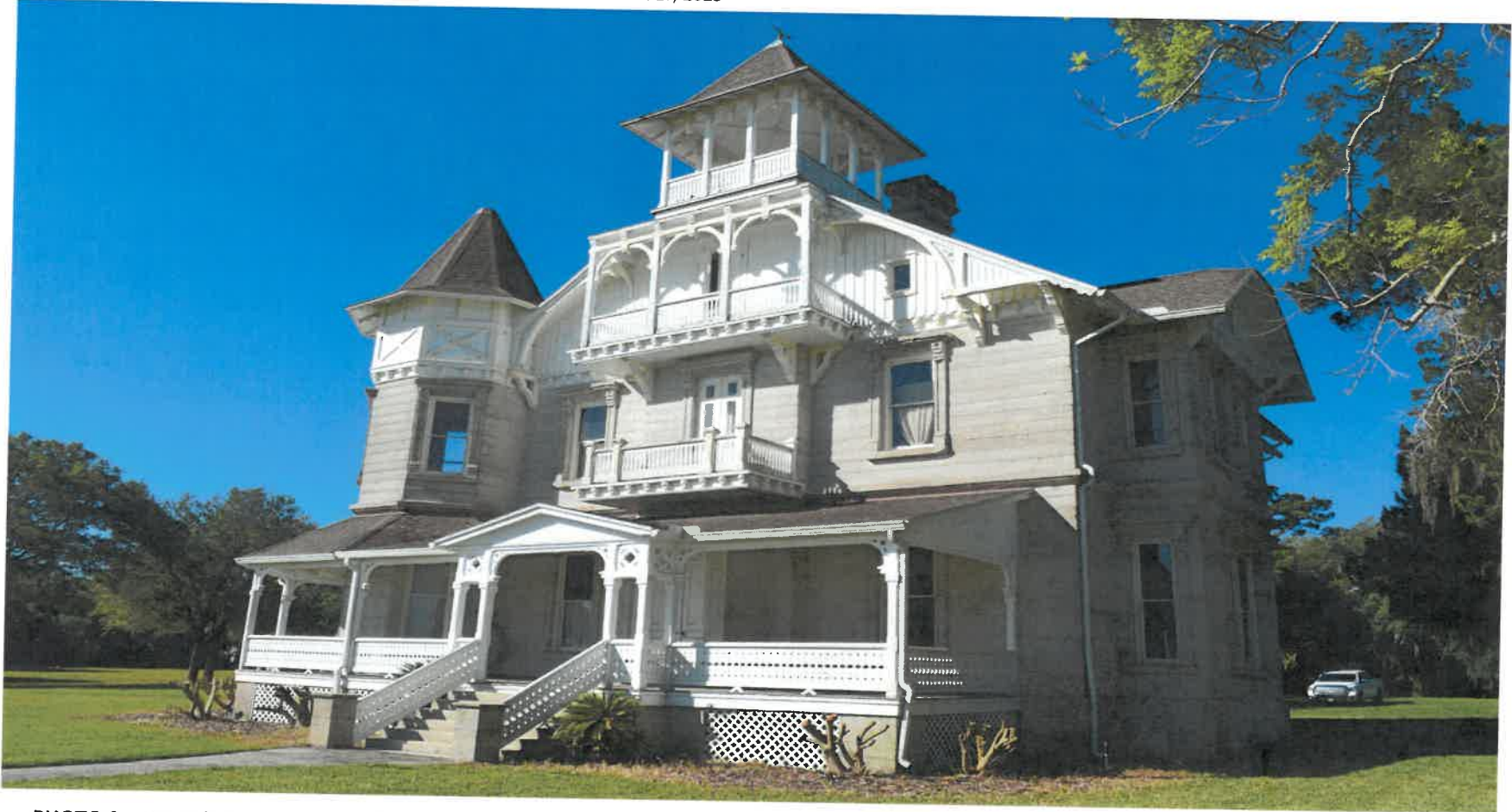
• PHOTO 8: MAIN (EAST) FAÇADE AND NORTH FACADE, CORNER TOWER AND EASTLAKE DETAILING, FACING WEST
