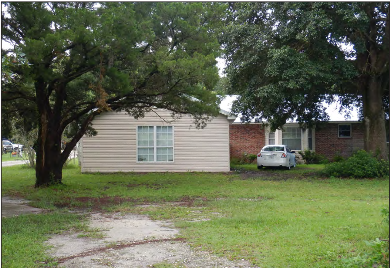
Figure 4.6. View of SJ07417, 6435 SR 16 HR.
