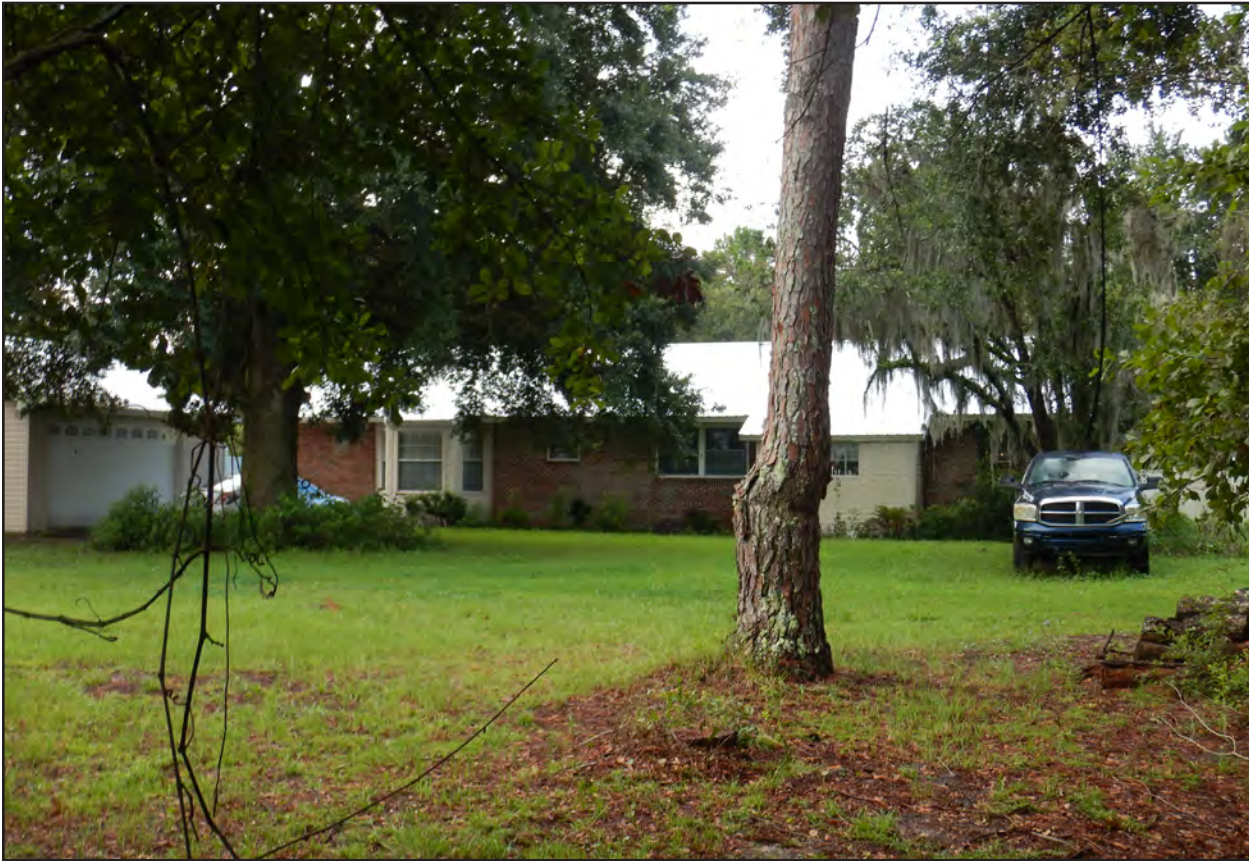
Figure 4.7. View of 6435 SR 16 HR.
