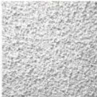
White Stucco on Concrete Masonry Units
