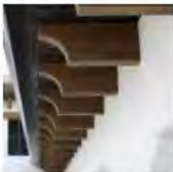
Decorative Rafter Tails
