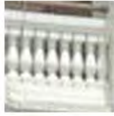
Cast Stone Balustrade
