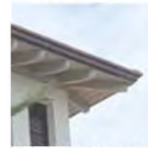
Wood Rafter Tail
