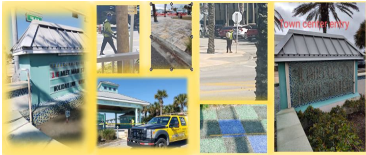
SJC helpful in repairing infrastructure
