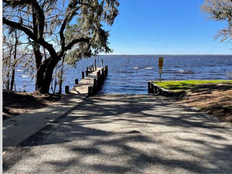
Riverdale Boat Ramp
